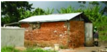
Goyavier water tank This CFTC-built cistern will provide 10 families with 8,000 litres of drinking water during the dry season.
